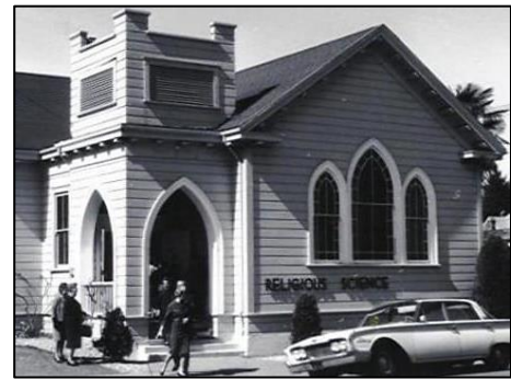
CHURCH BUILDING ON ORCHARD STREET
