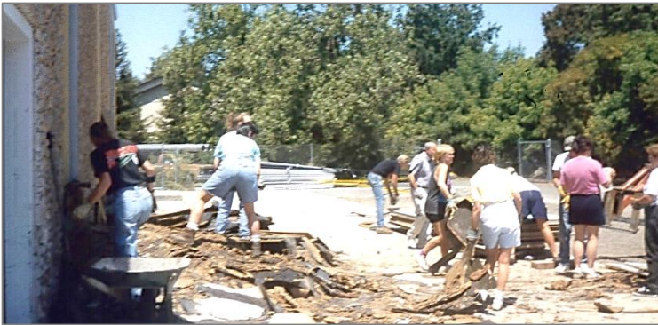
DEMOLITION AND CLEANUP BEGINS AT THE FORMER SKATING RINK
